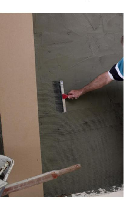
Made of light weight concrete which consist of polymers, cement, recycled aggregates, sand and pigments.
